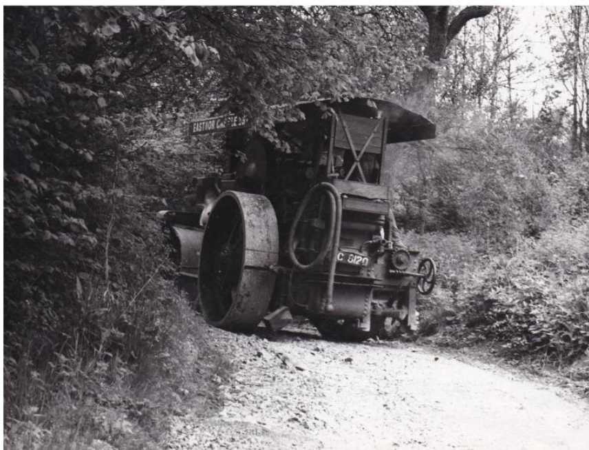
Fig. 2 Aveling & Porter No.14077 on more challenging work.
