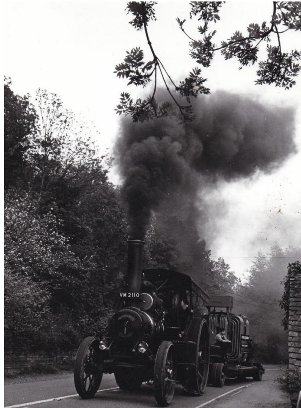
Fig.12 “ATLAS“ with trailer and concrete filled transformer.
